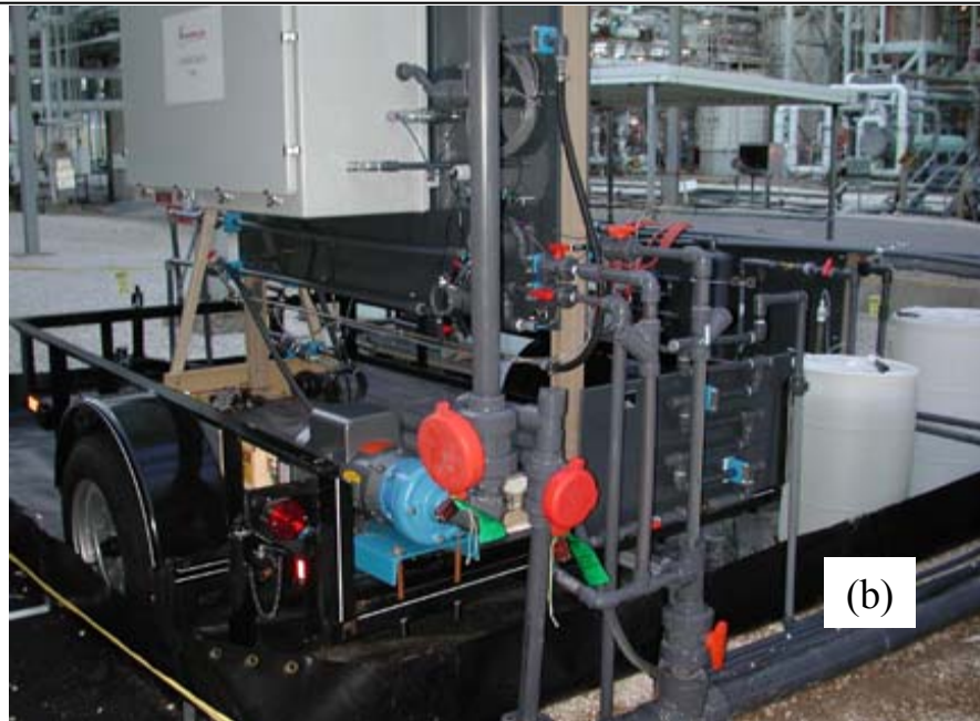
Figure 15. (a) Typical maximum localized corrosion rates of CMAS carbon steel probes measured in (b) a cooling water monitoring station of a chemical plant. Source: Ref. 86.
