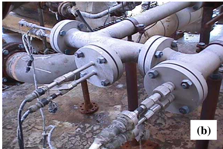
Figure 14. (a) Maximum localized corrosion currents of three alloys in (b) a pressurized stream of a chemical plant at elevated temperatures. Source: Ref. 79 and Ref. 83.
